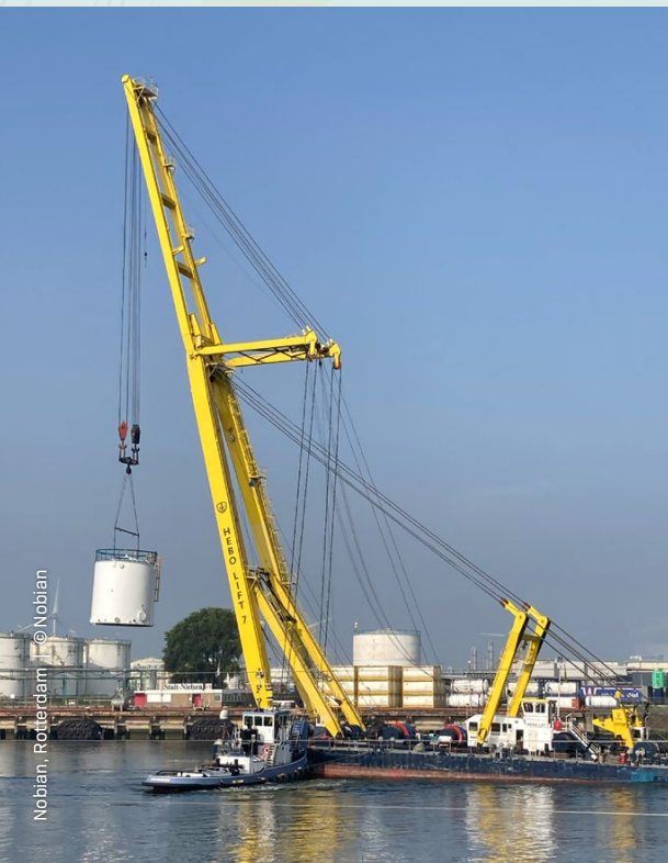
Installing the catholyte blowdown tank in Rotterdam.
