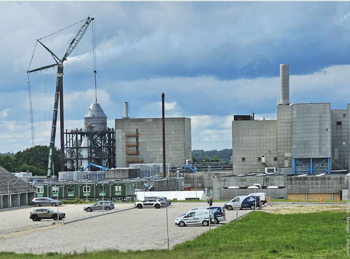
Hoisting the crystallizer into the steel structure at our Mariager site.
